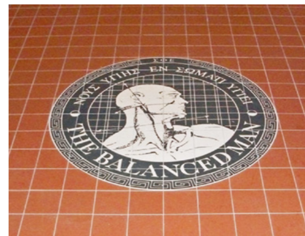
Logo printed black on white tiles then cut by water jet for precision. Tiled into a field of red 151mm squares. From sketch to finished foyer.
